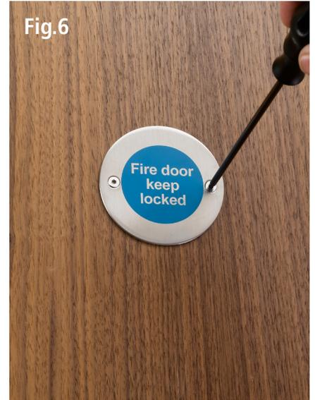
Allgood push / kick plates and signage are durable and require little maintenance. However, a frequent check should ensure that the items are firmly attached to the doors.
