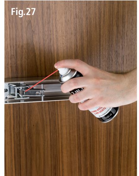
Panic hardware is extremely important in the event of a fire, so it is imperative that regular checks are undertaken to ensure that the device operates correctly.
