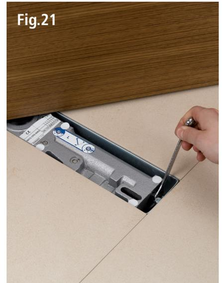
All Allgood floor spring mechanisms are sealed for life and require little maintenance. However, a frequent check should ensure that the door closes freely and positively into the frame.
